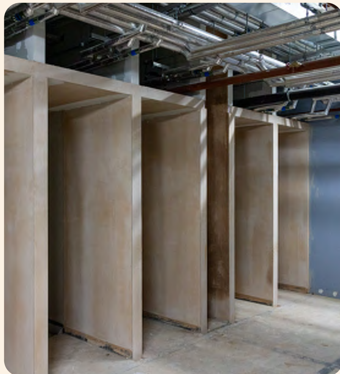
Shower cubicles on Basement -1
