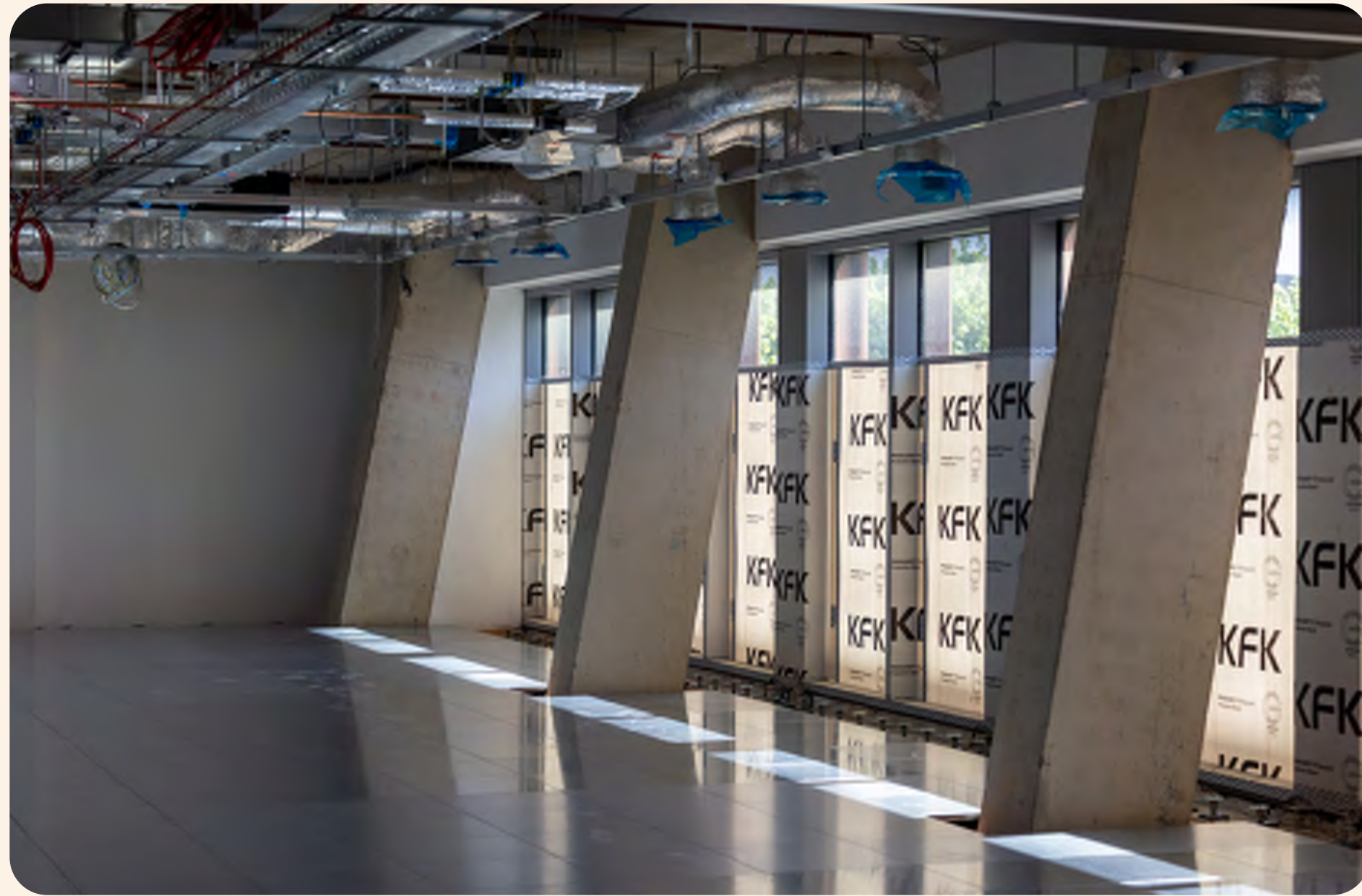
Raised access floor panels and second fix M&E on Level 2
