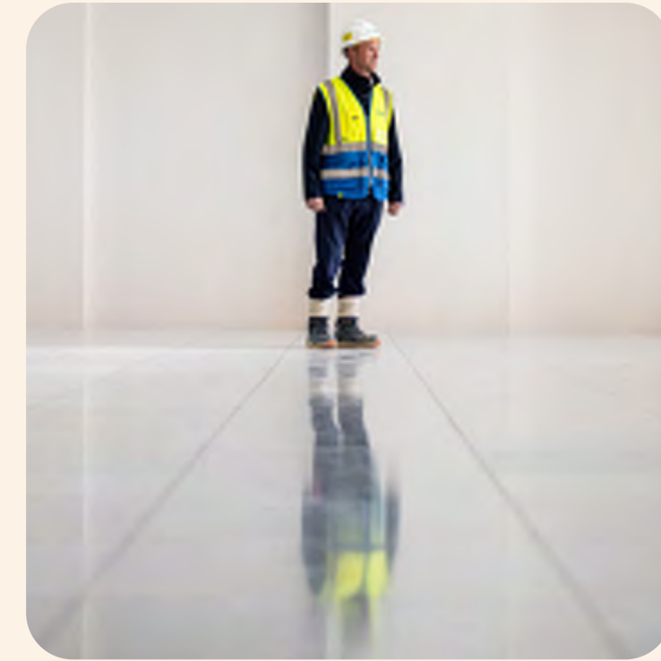
Raised access floor panels and painted walls on Level 2
