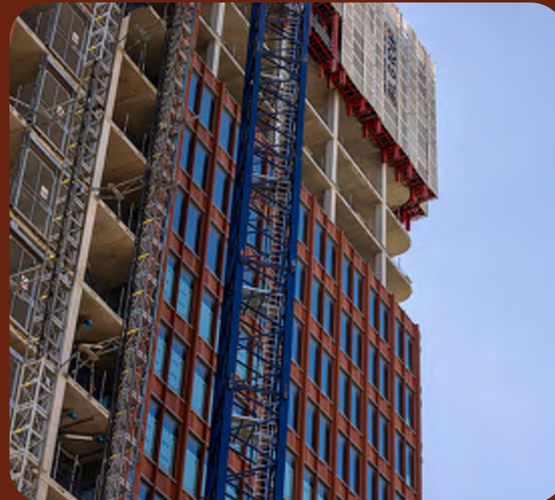
Façade panels up to Level 14
