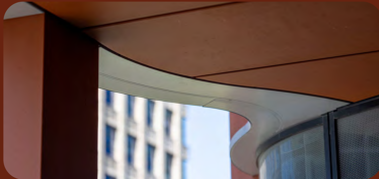
Terrace soffit on Level 3
