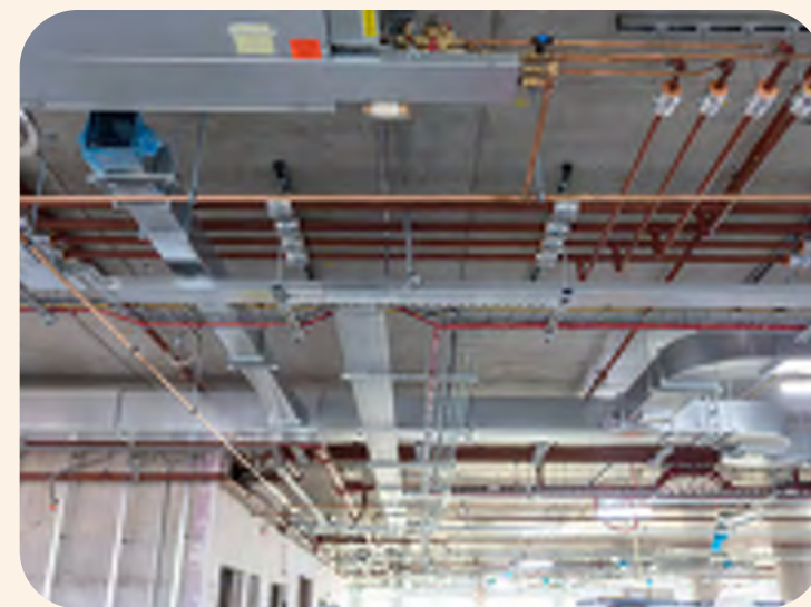
First fix M&E on level 6
