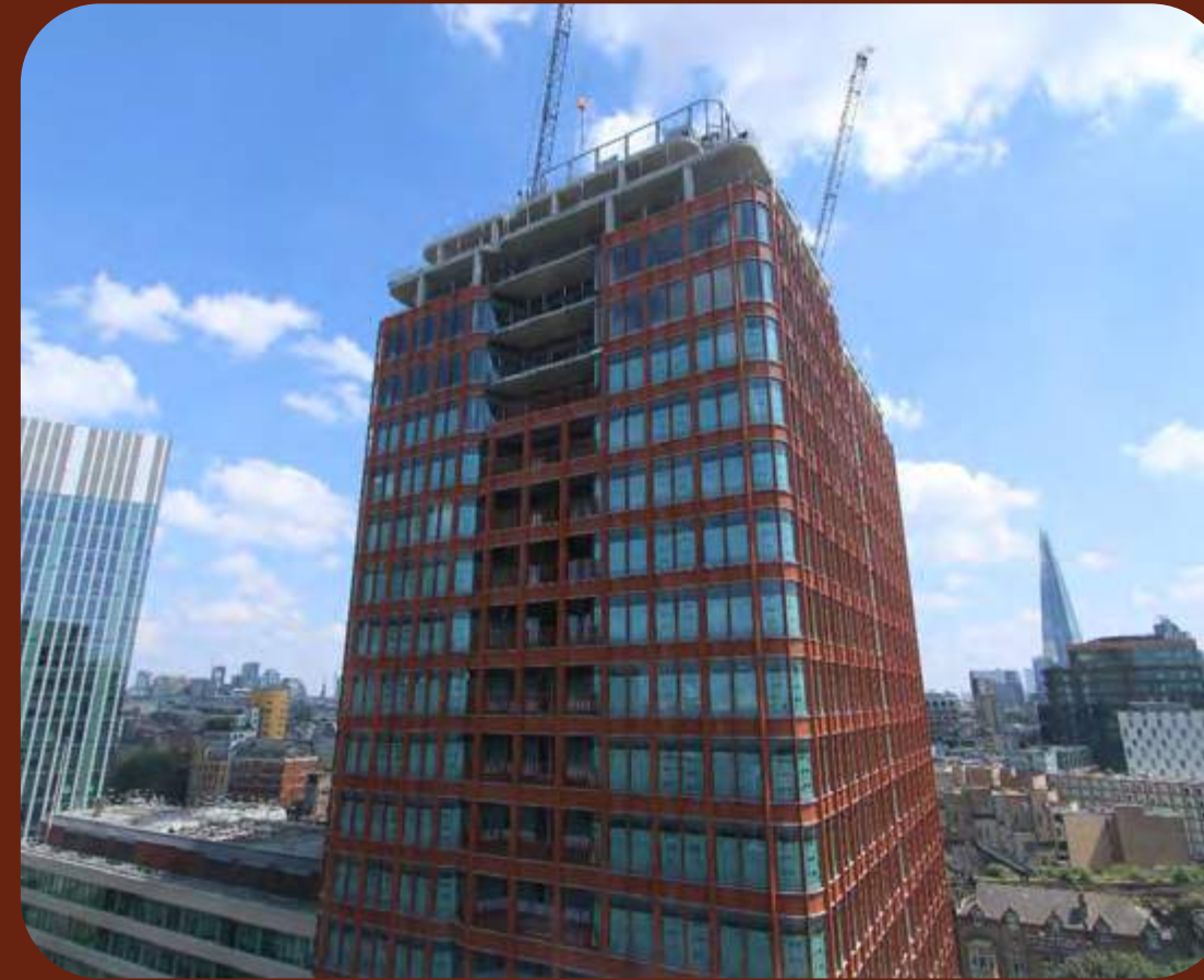
Façade installation up to Level 18
