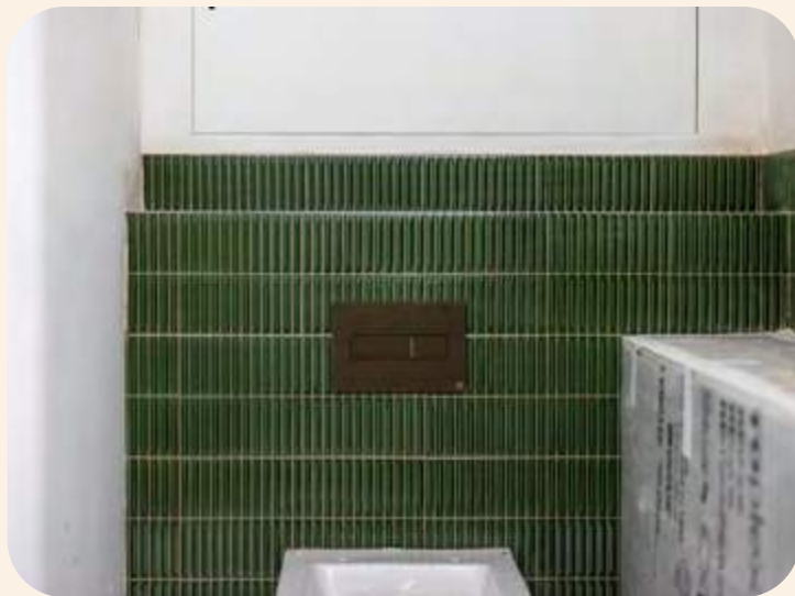
Level 3 super-loo tiling & sanitary-ware
