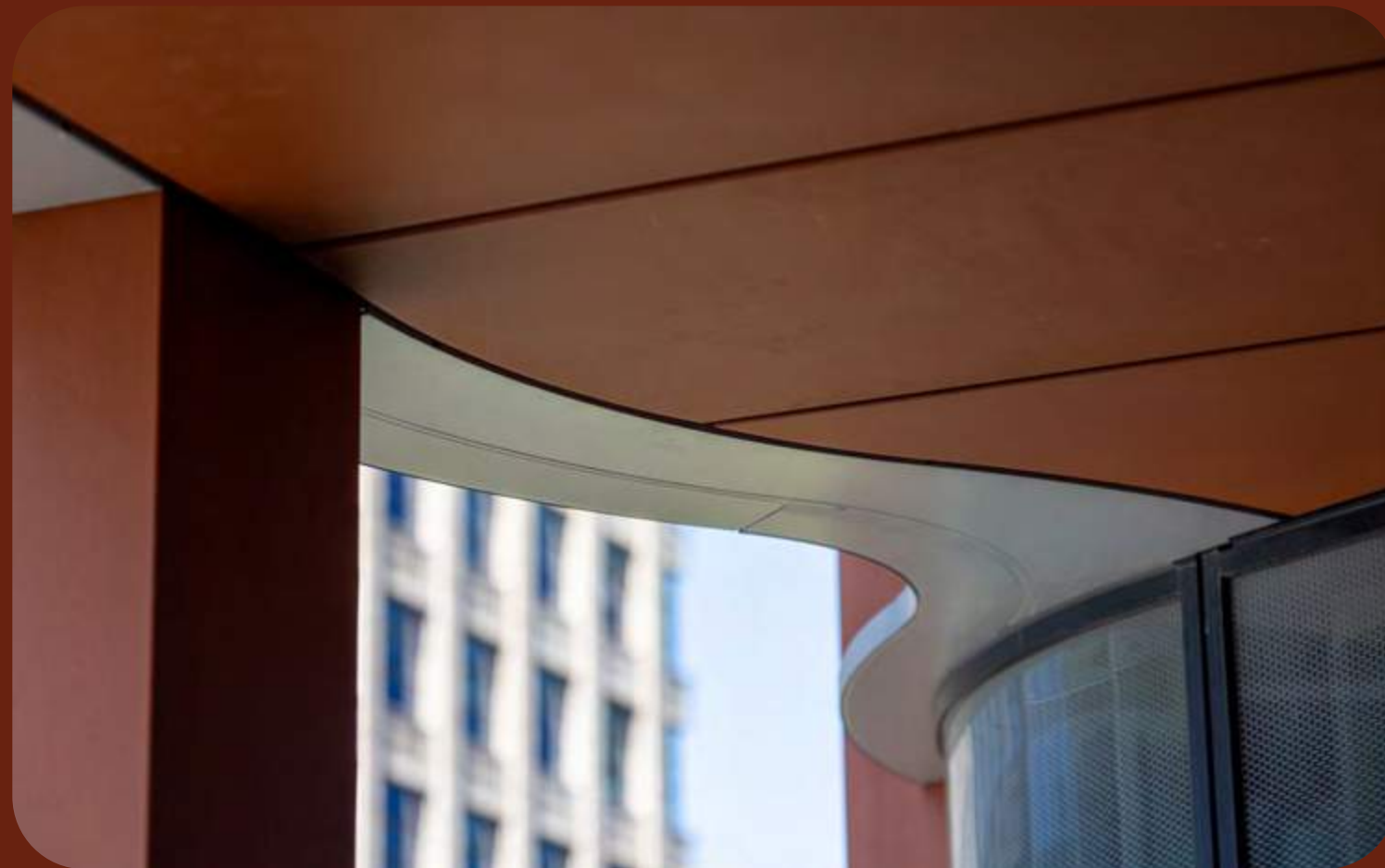
Terrace soffit on Level 3
