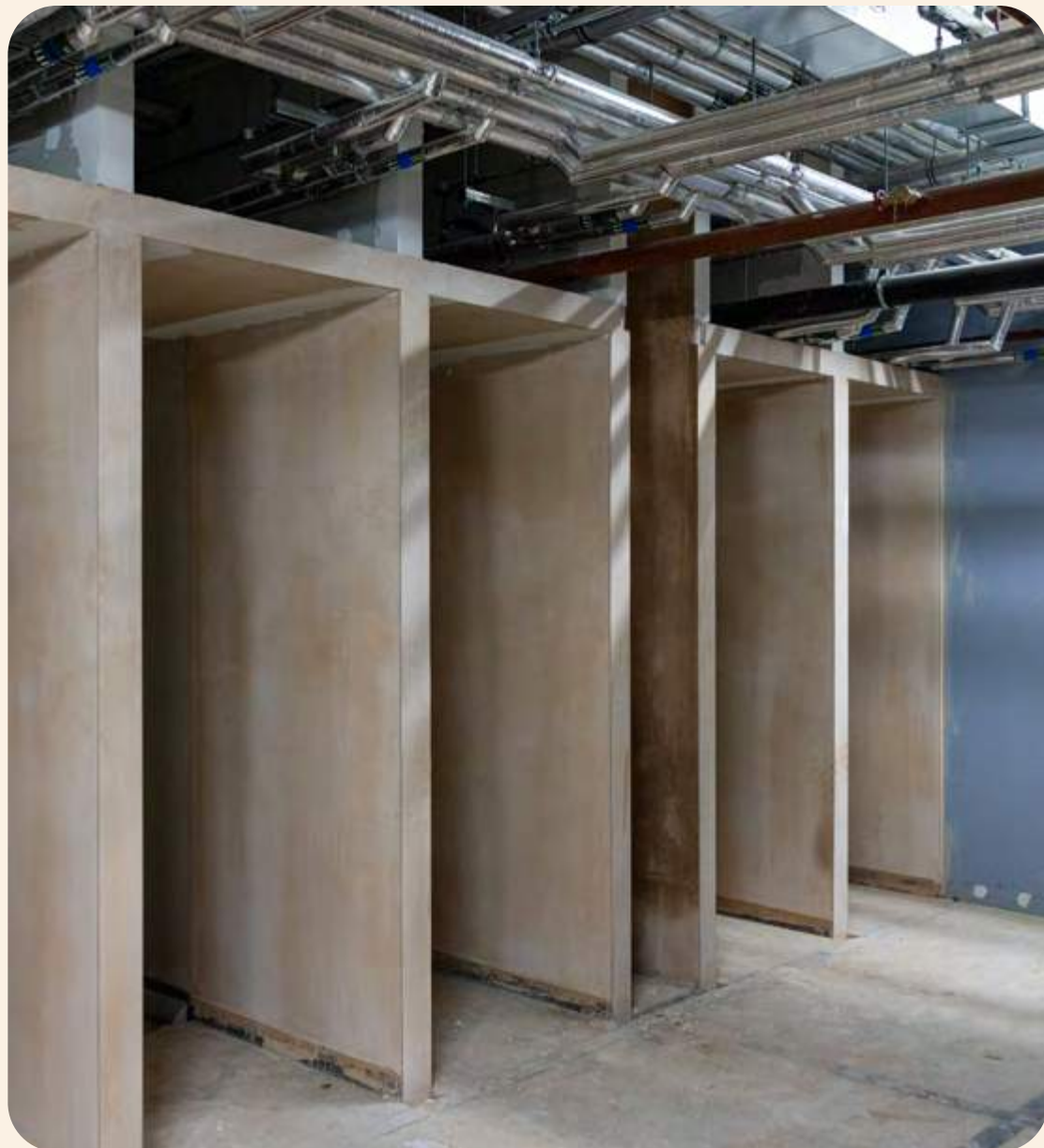
Shower cubicles on Basement -1
