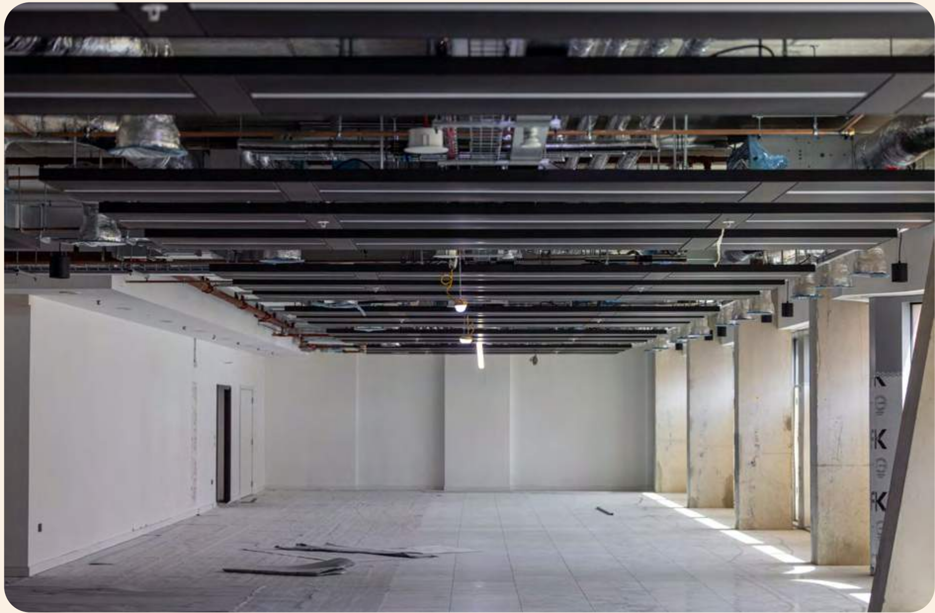
Raised access flooring & Kreon raft ceilings on Level 3
