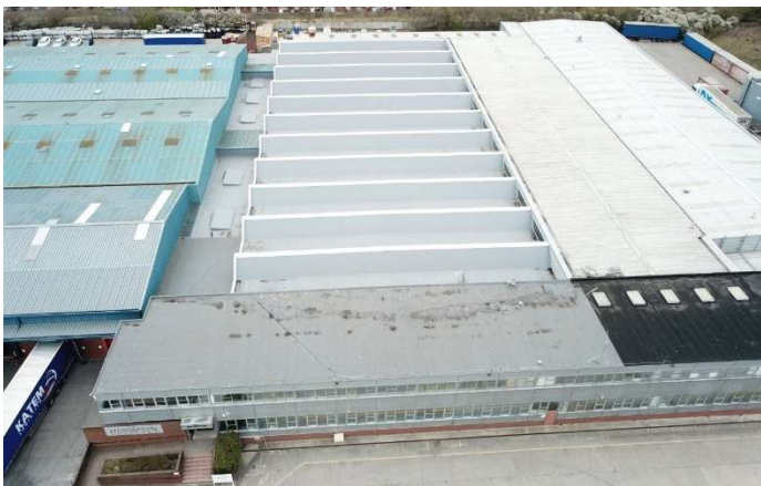
New roof covering on Unit 2 (2025).
