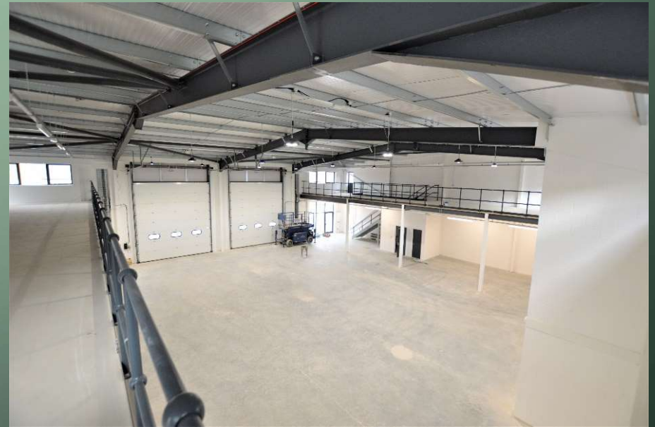
Under floor heating with air source heat pumps, intelligent LED lighting, mezzanine, shower and toilets
