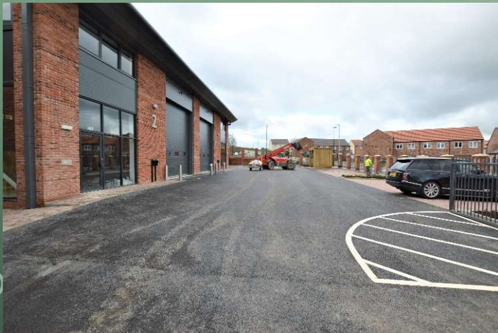
Anti-ram bollards and 2 electric chargers per unit
