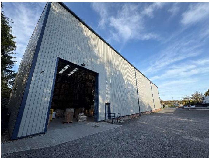
Unit 2 High Bay Warehouse
