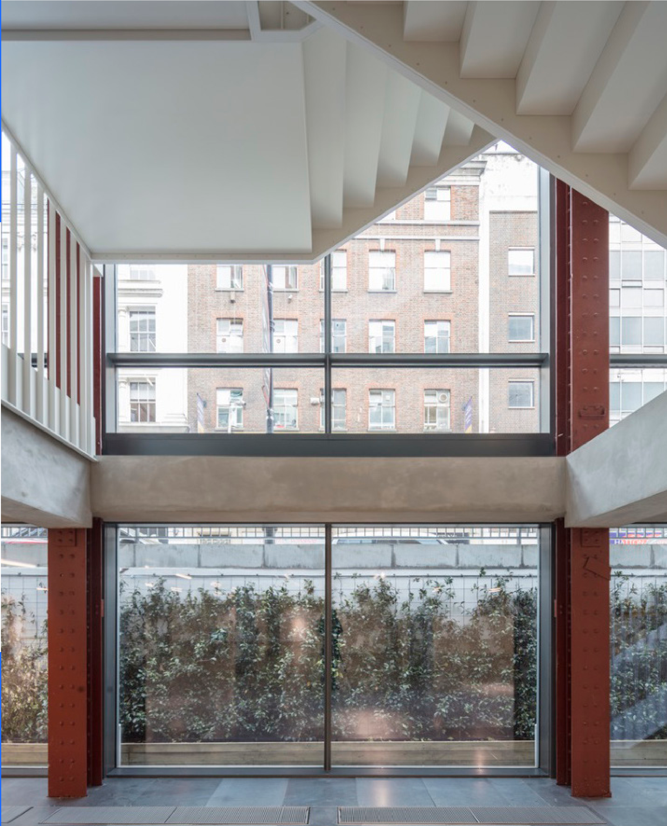
Lower ground floor glazed elevation (indicative photos)
